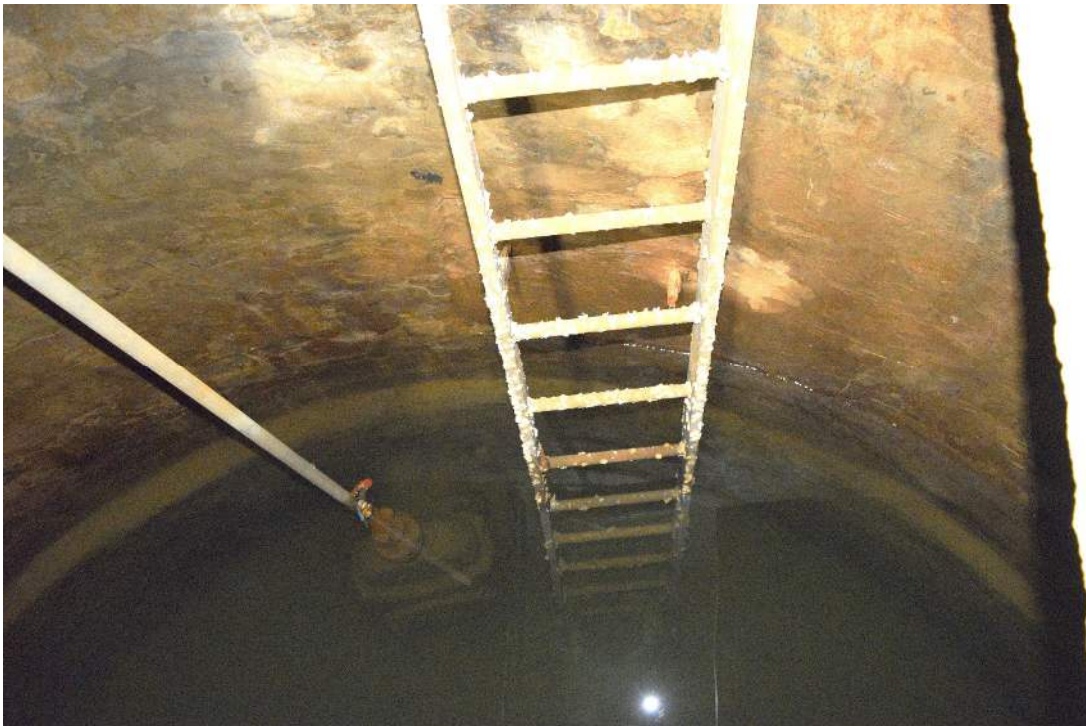
FIGURE 36: LOOKING INTO STONE LINED WELL
