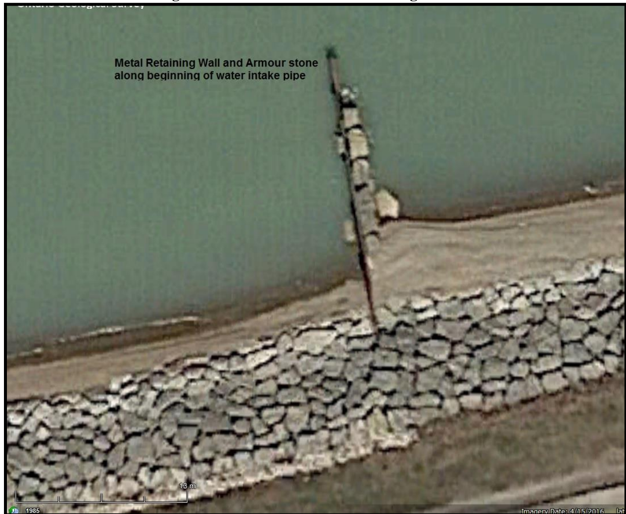
Figure 4: Metal Sheet Wall at Existing Intake
