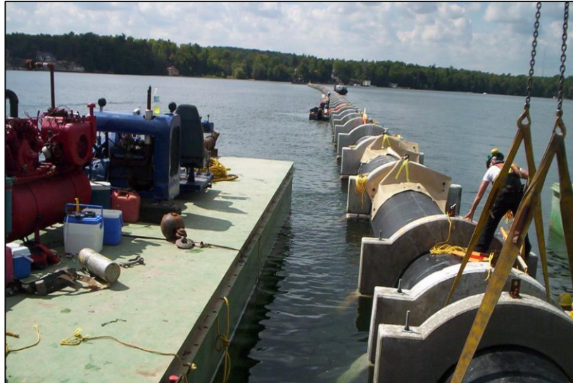
Installation of intake pipeline with ballast to prevent pipeline from floating
