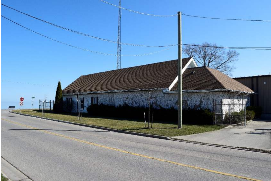
FIGURE 12: SOUTHEAST EXPOSURE, FACING NORTHEAST
