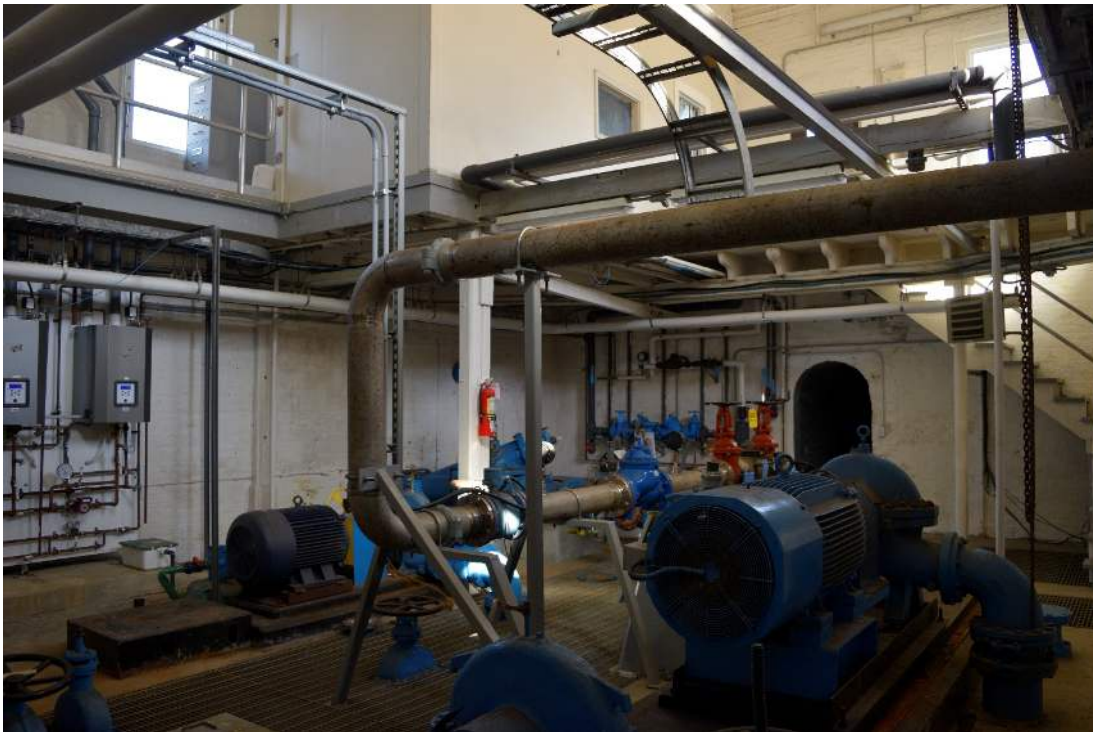
FIGURE 32: LOWER LEVEL, FACING NORTH
