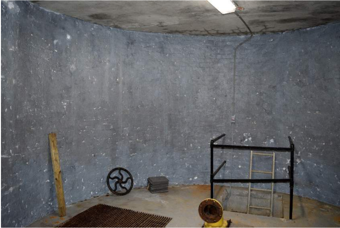
FIGURE 35: WELL VAULT FACING NORTH
