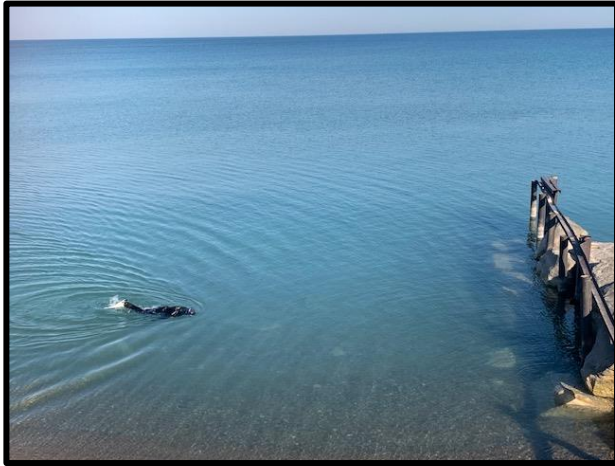
Image 7: Snorkel survey near intake and metal retaining wall
