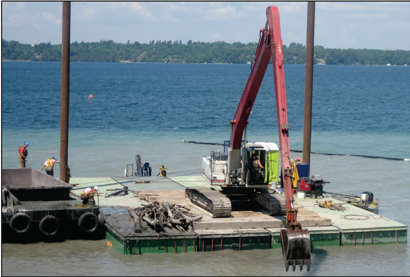
Excavation of marine trench with floating dredging equipment
