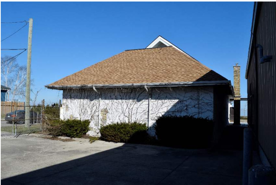
FIGURE 15: SOUTHEAST CORNER OF STRUCTURE, NOTE PROXIMITY OF ADJACENT STRUCTURE PREVENTING FULL DOCUMENTATION OF EAST FACE
