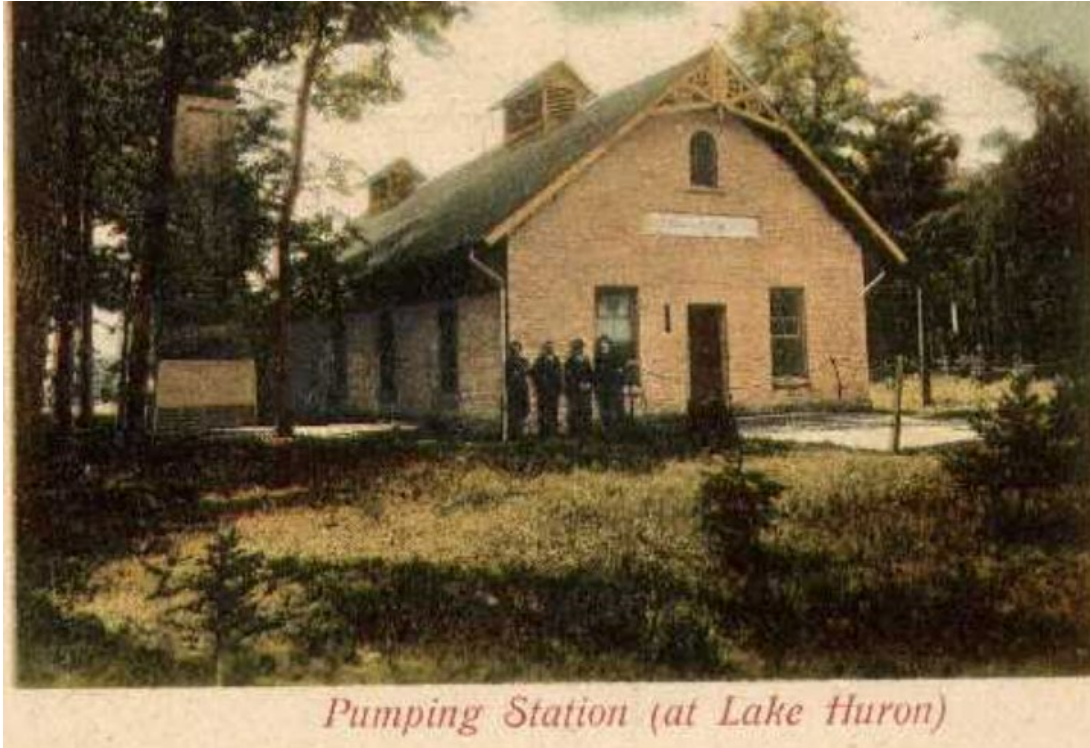
Figure 1: Undated colorized historic image of 'Petrolia Water Works', image from Petroliaheritage.com
