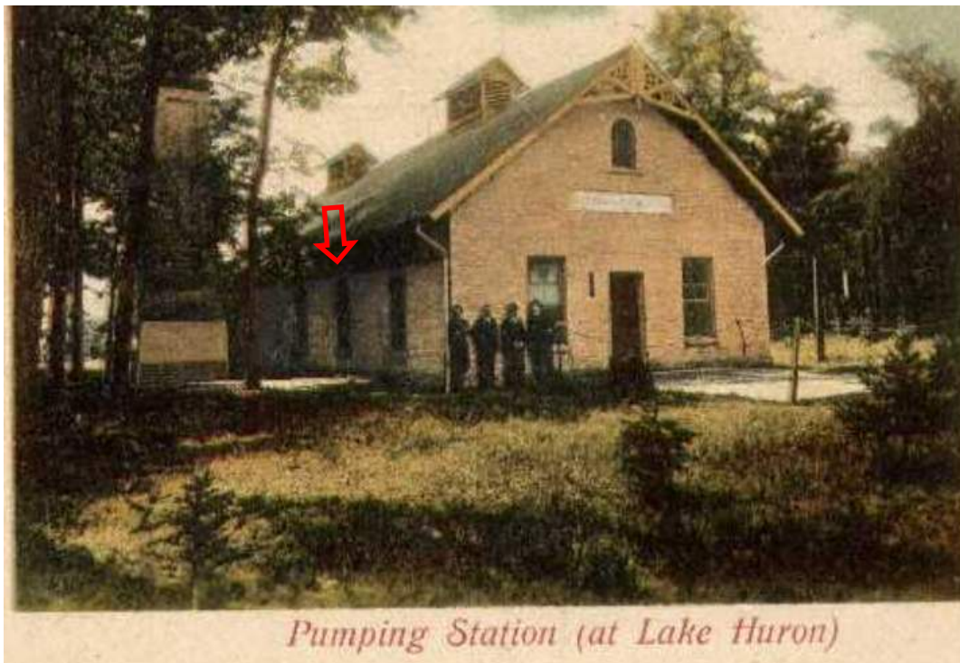
FIGURE 2: UNDATED COLORIZED HISTORIC IMAGE OF 'PETROLEA WATER WORKS' IMAGE FROM PETROLIAHERITAGE.COM, RED ARROW INDICATES ORIGINAL WINDOW OPENING THAT WAS ALTERED TO FORM EQUIPMENT EGRESS DOOR
