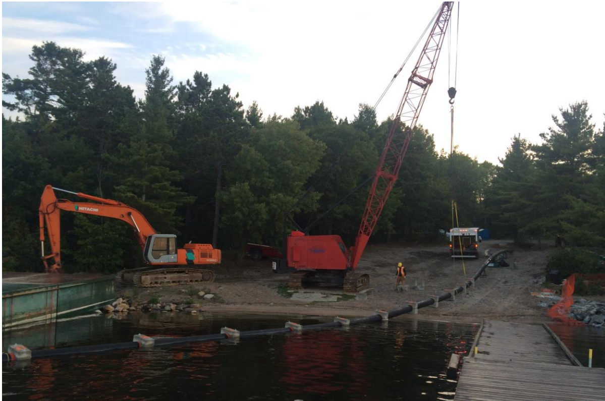
Figure 2-7: Example onshore installation of intake pipeline
