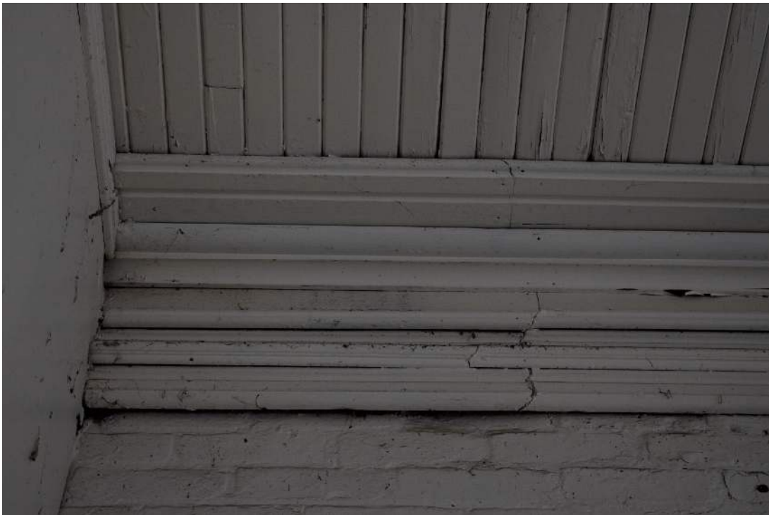
FIGURE 40: EXAMPLE OF ORIGINAL MILLWORK
