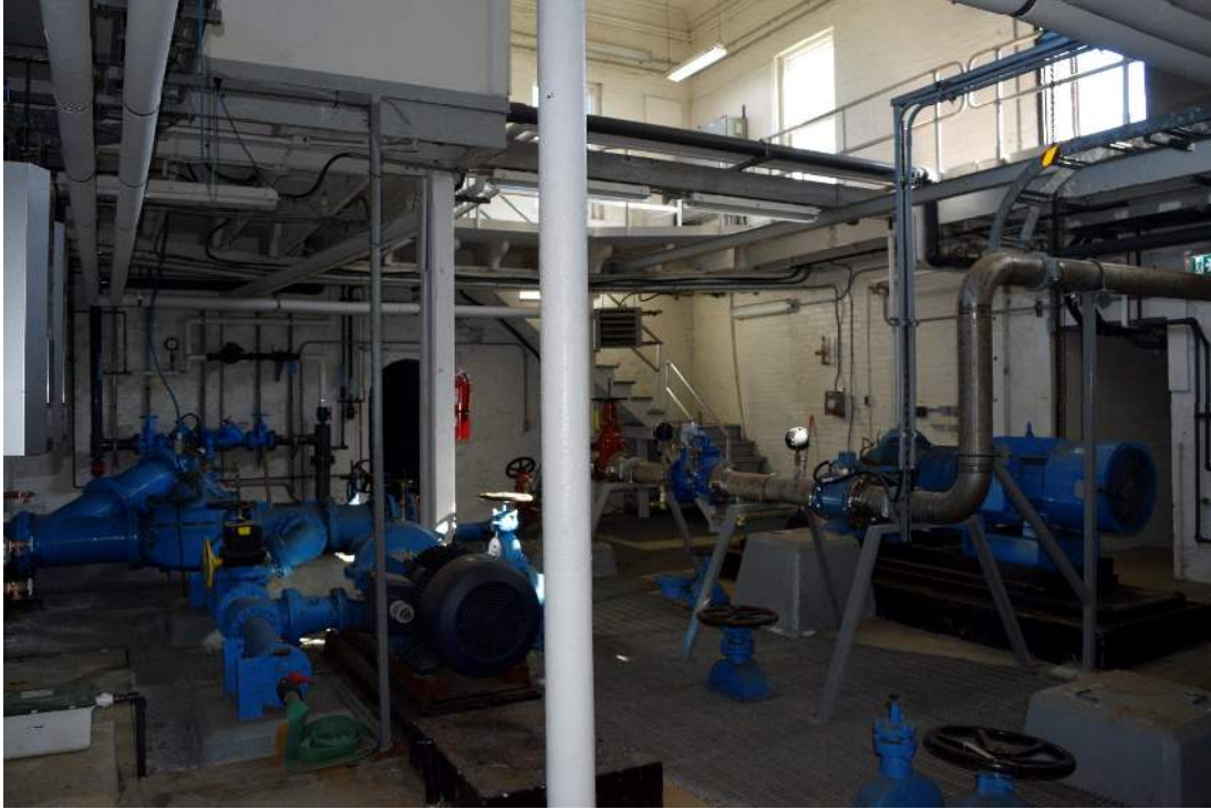
FIGURE 33: LOWER LEVEL FACING SOUTH
