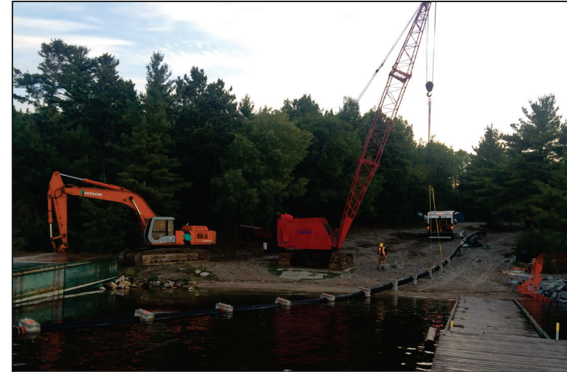
Onshore installation of intake pipeline
