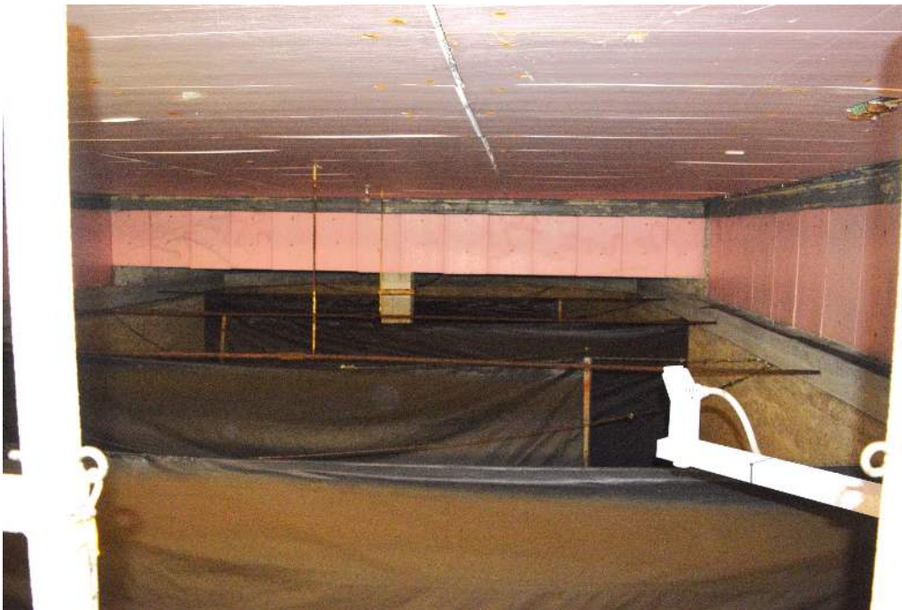
FIGURE 38: LOOKING SOUTH OVER THE WATER SETTLING TANKS
