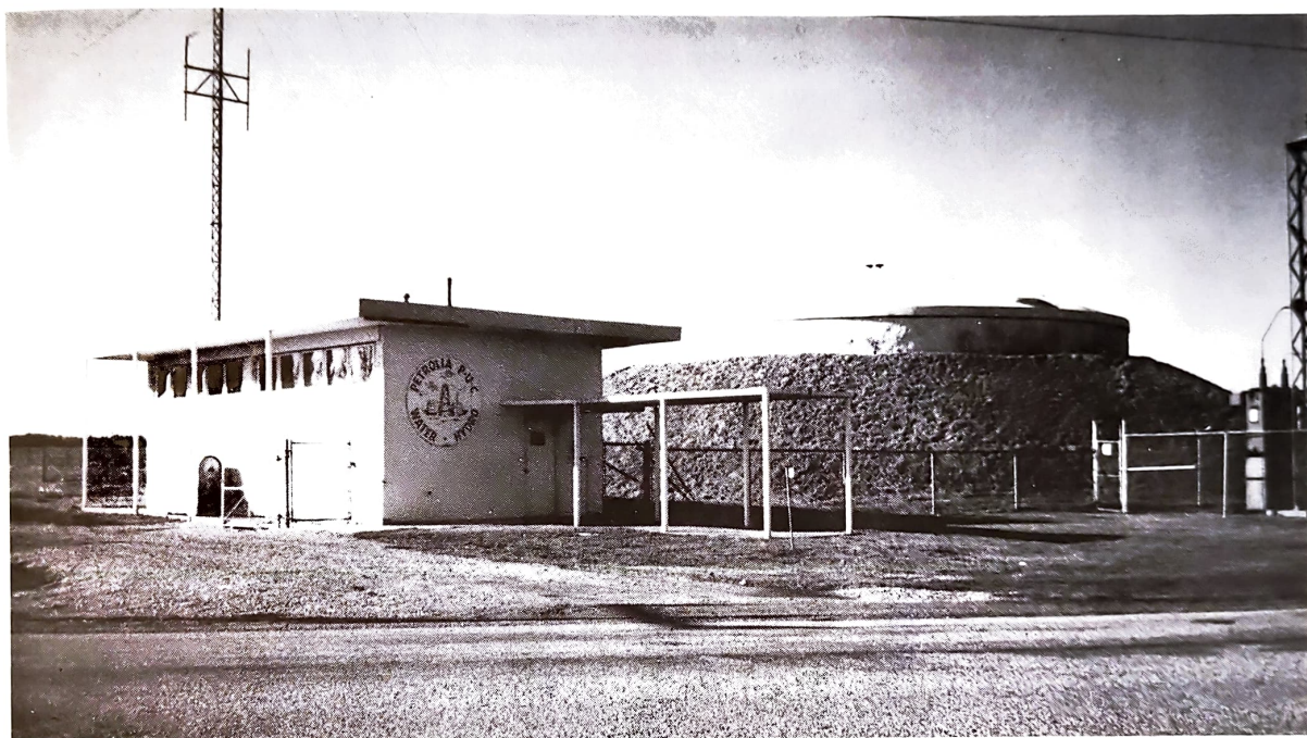
Reservoir & Pumping Station
