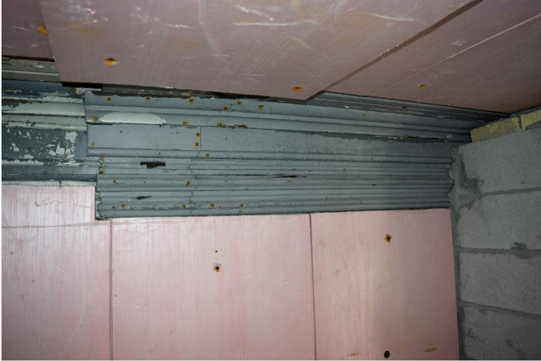
FIGURE 39: ORIGINAL MILLWORK AS SEEN IN NORTHWEST CORNER OF WATER SETTLING TANK ROOM
