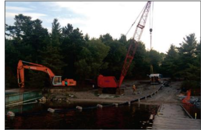
Onshore installation of intake pipeline
