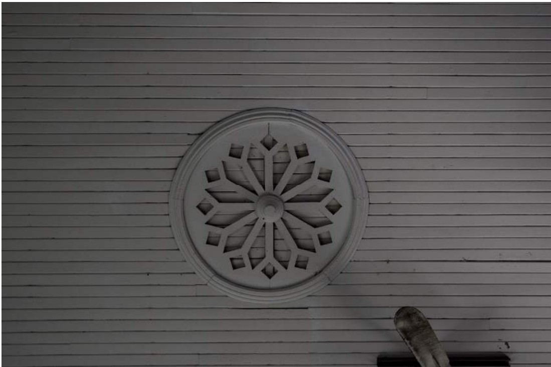
FIGURE 42: CLOSEUP OF CEILING MEDALLIONS
