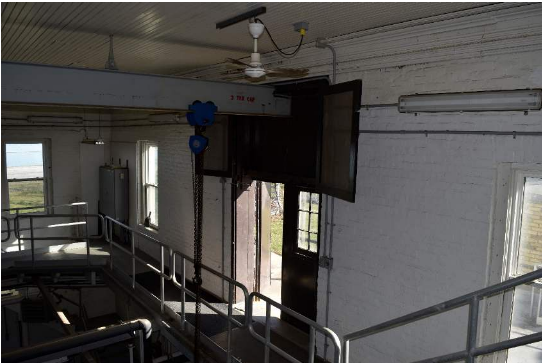
FIGURE 28: OVERSIZED HEAVY EQUIPMENT EGRESS WITH ASSOCIATED HOIST
