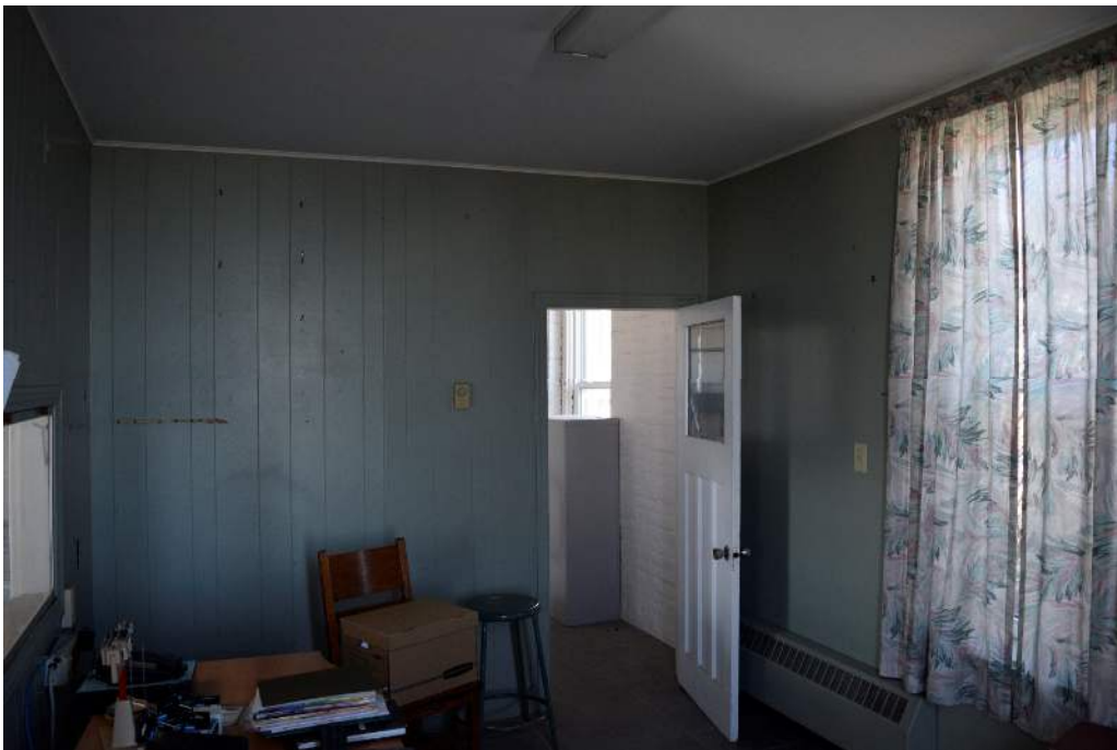
FIGURE 26: OFFICE LOCATED IN NORTHWEST CORNER OF STRUCTURE, FACING SOUTH
