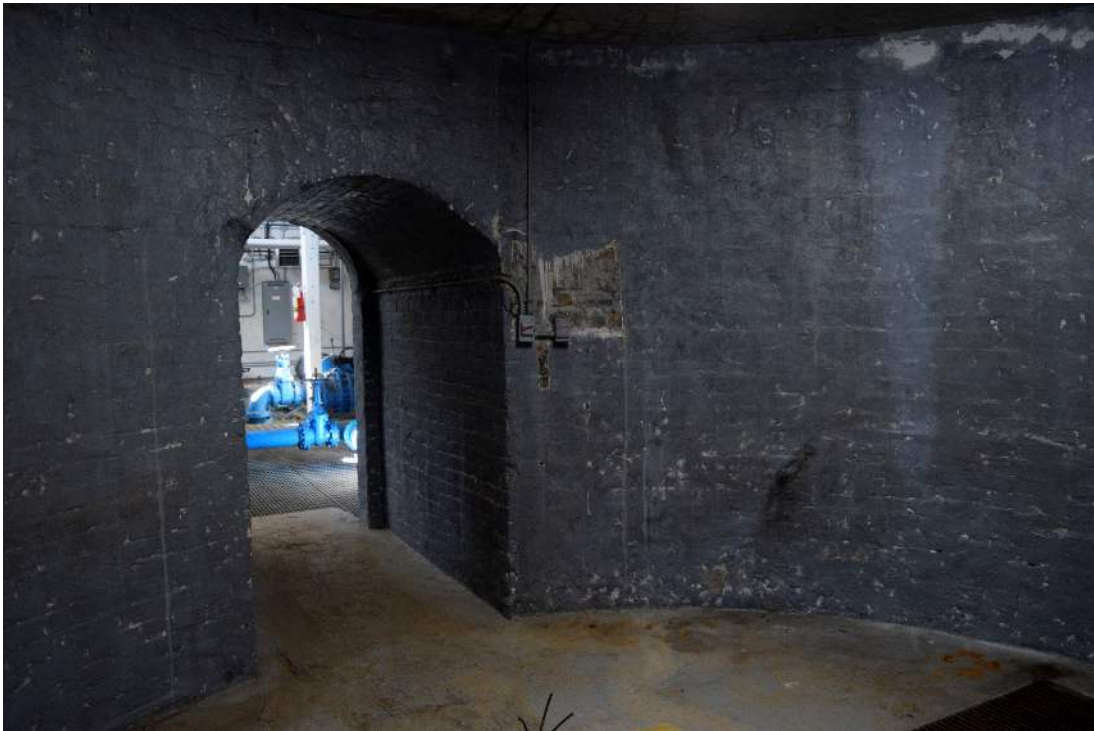
FIGURE 34: WELL VAULT AND CONNECTING PASSAGE, FACING SOUTH
