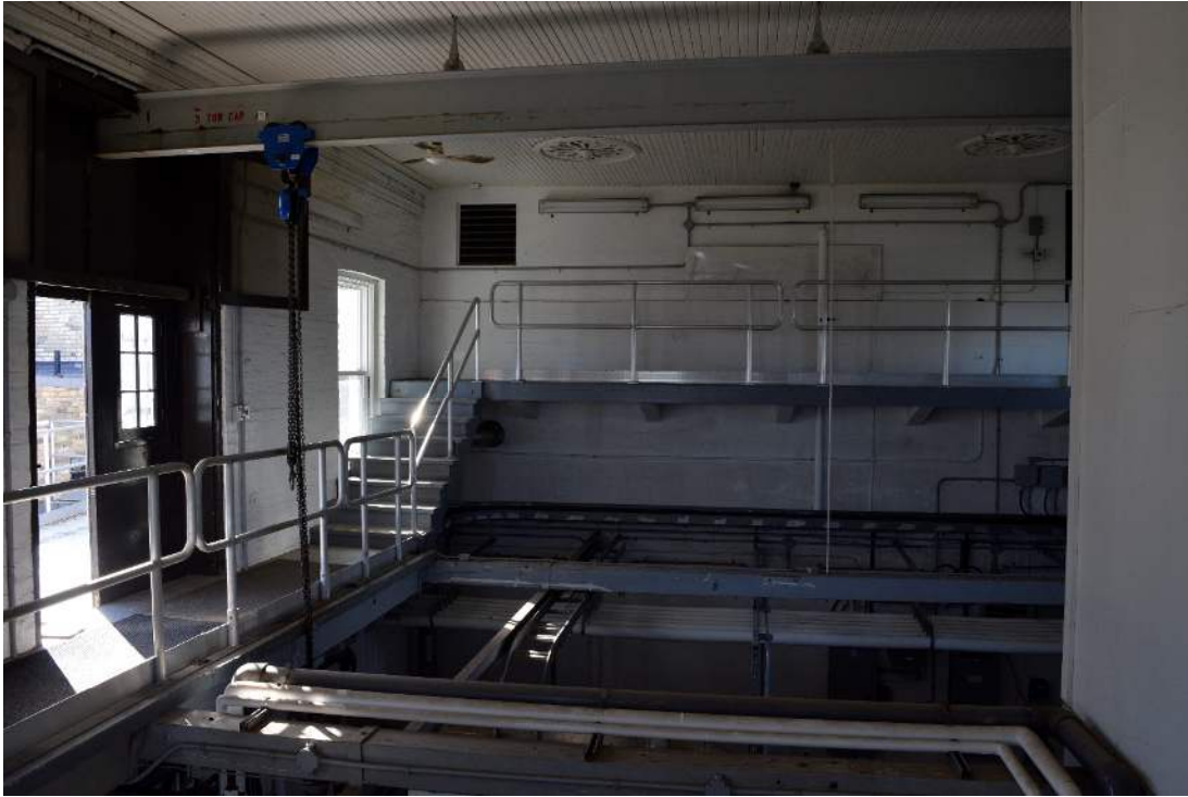
FIGURE 29: LOOKING SOUTH ALONG EAST WALL OF STRUCTURE, FACING SOUTH
