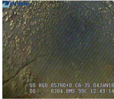
Figure 5-6: Cracked Intake
