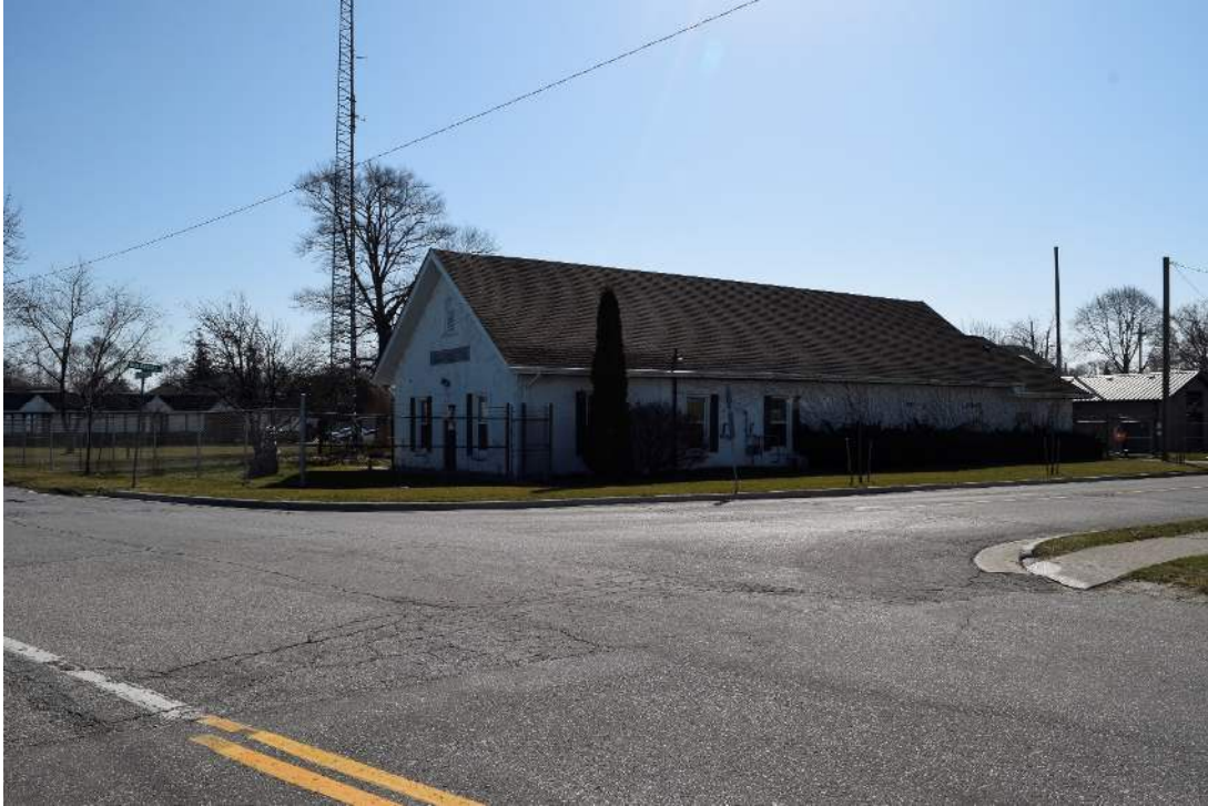
FIGURE 10: NORTHWEST EXPOSURE, FACING SOUTHEAST, INTERSECTION OF OLD LAKESHORE ROAD AND WATERWORKS ROAD IN FOREGROUND
