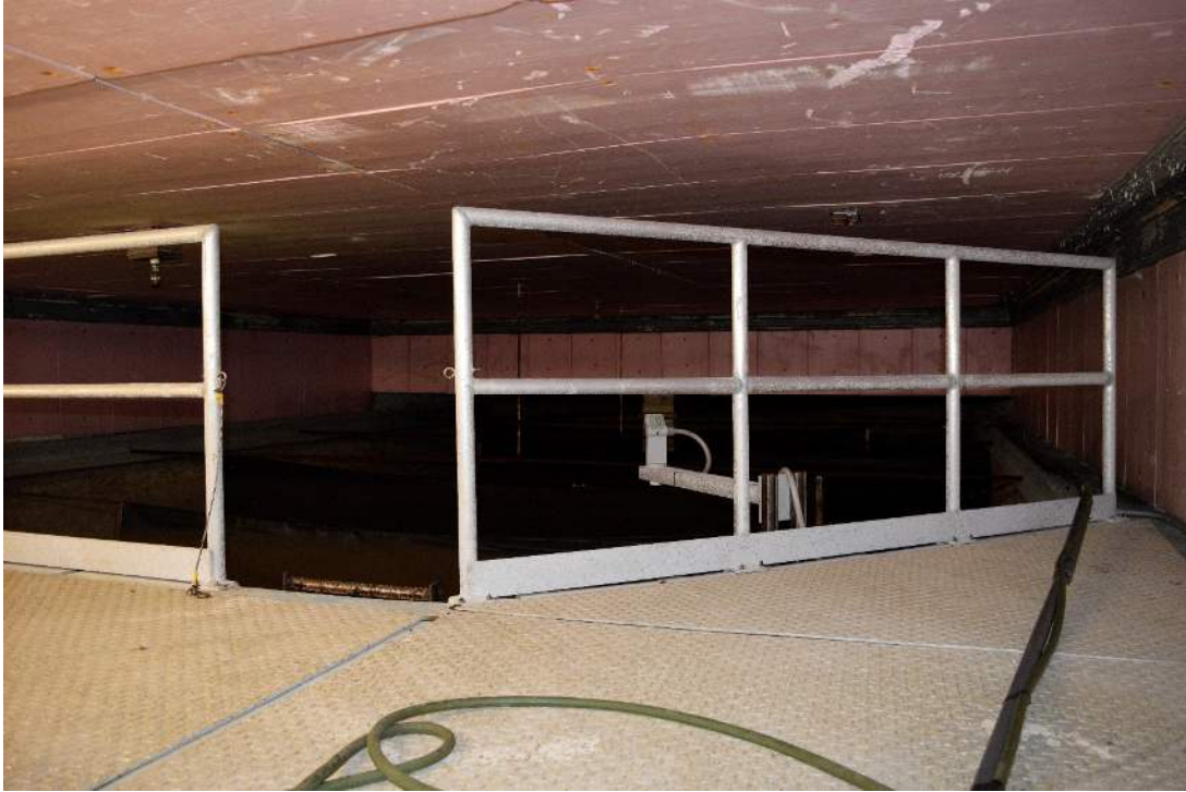
FIGURE 37: CATWALK ON NORTH END OF WATER SETTLING TANKS, FACING SOUTH
