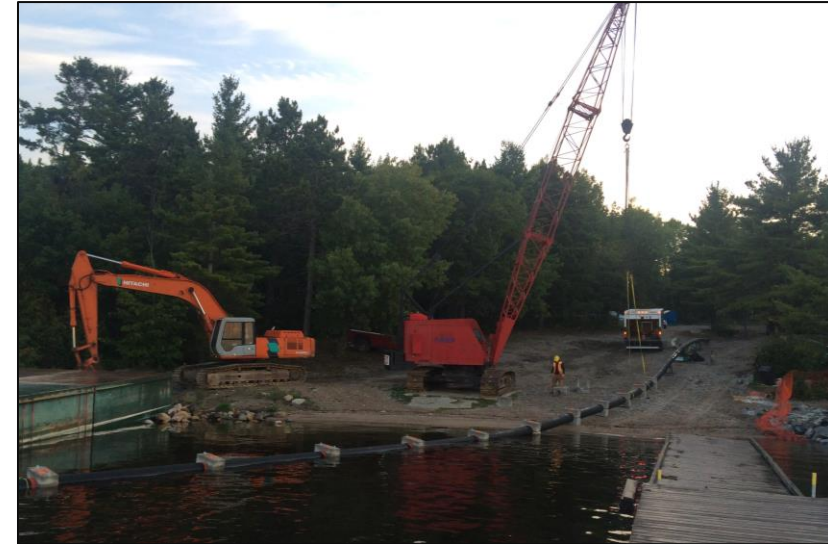
Onshore installation of intake pipeline
