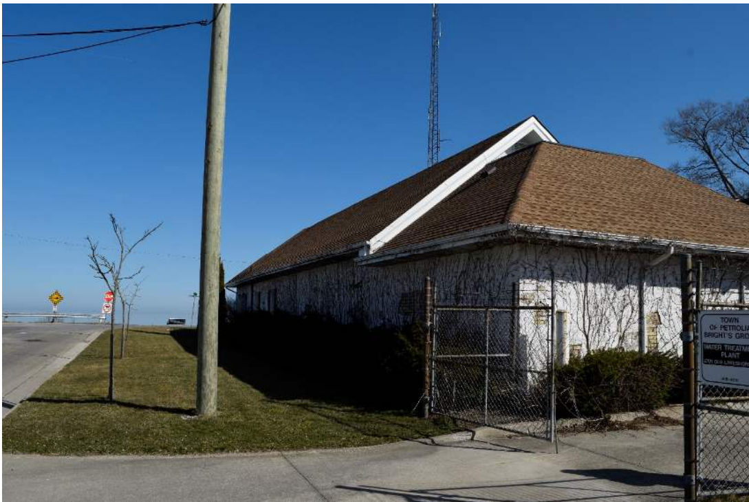
FIGURE 13: SOUTHEAST EXPOSURE, HIGHLIGHTING THE TRANSITION FROM GABLE ROOF LINE TO TRUNCATED HIP ROOF ON SOUTH END OF STRUCTURE
