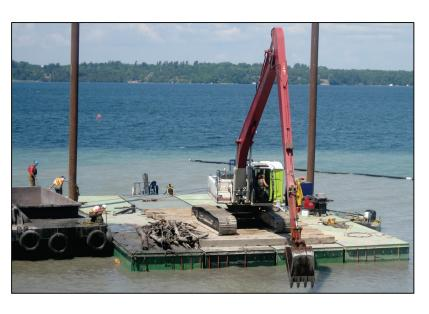
Excavation of marine trench with floating dredging equipment
