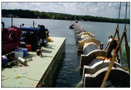
Installation of intake pipeline with ballast to prevent pipeline from floating
