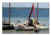
Excavation of marine trench with floating dredging equipment
