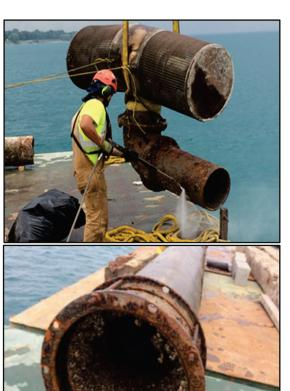
Photos taken of intake screen, pipe cut-out section, zebra mussel infestation, pipeline crack near the shoreline.
