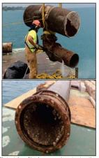
Photos taken of intake screen, pipe cut-out section, zebra mussel infestation, pipeline crack near the shoreline.
