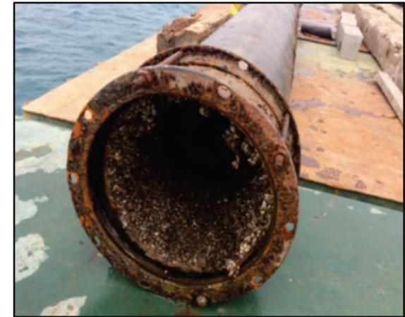
Photos taken of intake screen, pipe cut-out section, zebra mussel infestation, pipeline crack near the shoreline.
