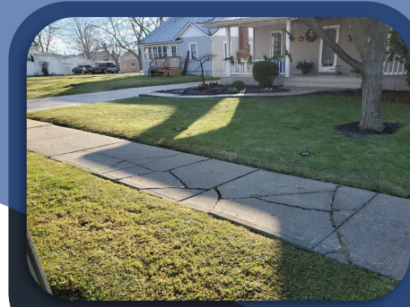
Cracking
