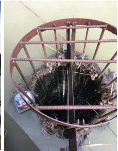
Existing Online Pond. Looking north from along retaining wall (left insert). Existing 600 mm CSP vertical pipe outlet (right insert).
