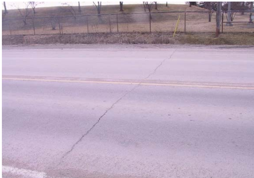
Transverse /Thermal cracking
